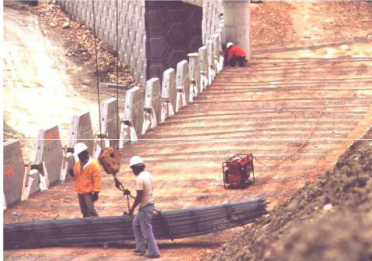
Galvanized metal strips are laid out behind the wall.
